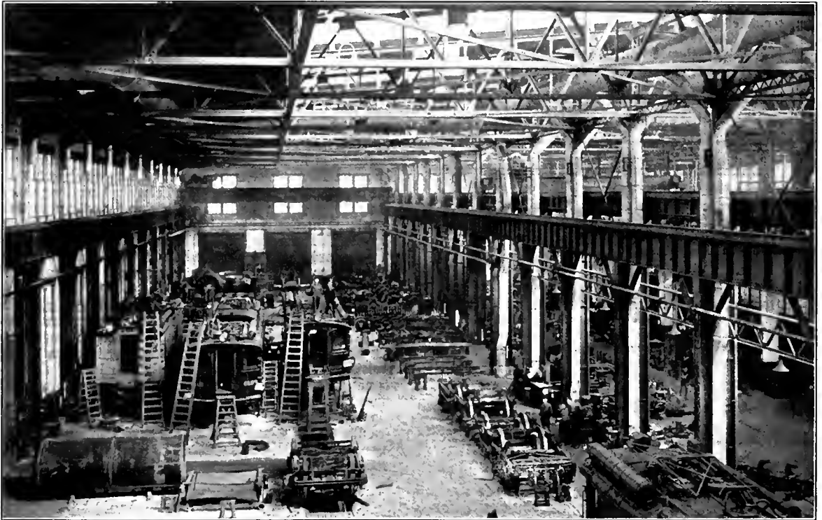
Fig. 2—General View of Erecting Shop for Electrical Equipment
